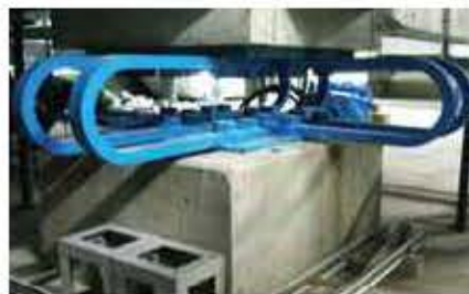
U型鋼材ダンパー U-shaped steel dampers
