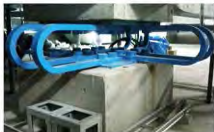
U型鋼材ダンパー U-shaped steel dampers
